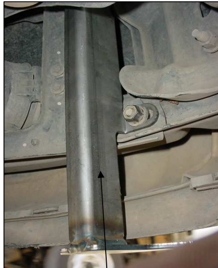
Installed main bracket, picture driver side.
